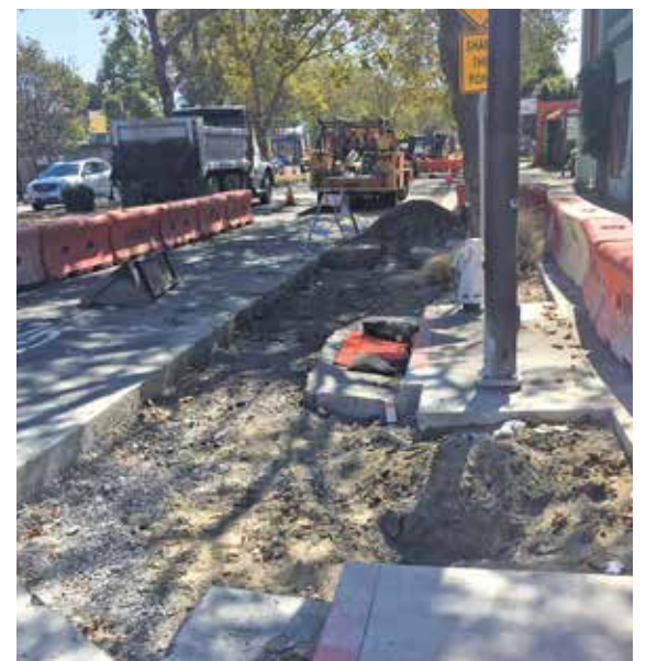
Replacing concrete surfaces with landscaping that collects runoff helps prevent contaminants from entering the Bay.
