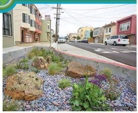
Planted bulb-outs and rain gardens constructed on a nine-block stretch of San Francisco's Holloway Street now provide a way of keeping stormwater out of the sewer system by capturing it upstream.
