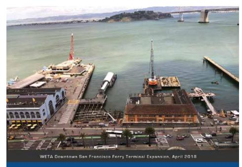
By April 2018, above-water construction was well underway. Placement of the cast-in-place concrete deck is progressing north and into the lagoon. All along the way and into the lagoon, temporary scaffolding and walkways are set up for the crew to build formwork and prepare for concrete pours.
