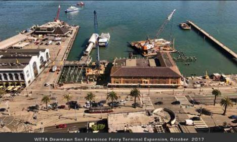
By October 2017 preparation of the site for above-water construction was nearly complete. Pier 2 had been demolished, the ferry terminal turning basin had been dredged and 154 large diameter steel pilings were installed, which are the foundation for the 35,000 square foot concrete deck expansion and new pedestrian bridge.
