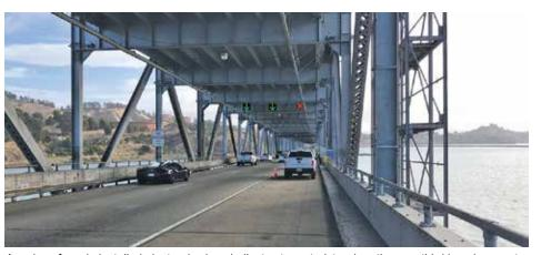
A series of newly-installed electronic signs indicates to motorists when the new third lane is open to traffic. Green arrows indicate open lanes and a red X indicates a closed lane.
