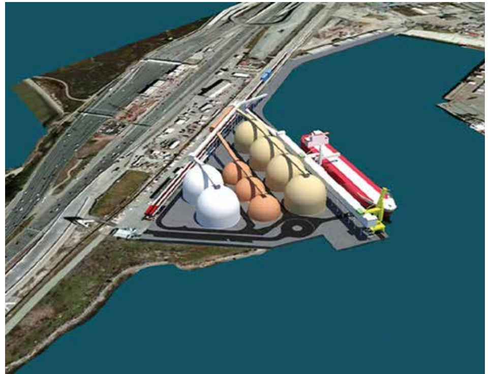
The TLS proposal calls for domed coal storage and covered railcars that, supporters say, will significantly reduce dust and pollution.
