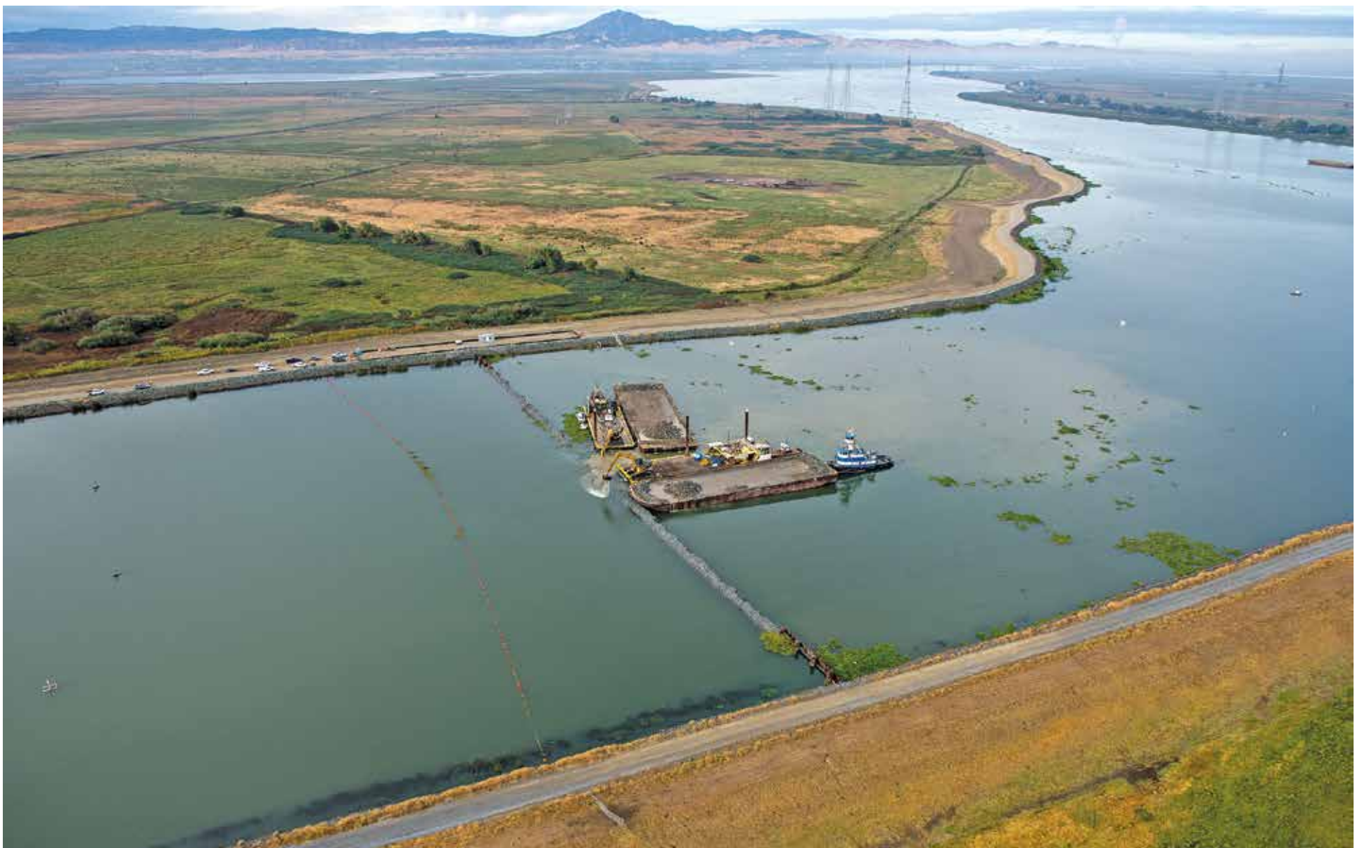
The salinity barrier was an essential part of the California Department of Water Resources' strategy to maintain good water quality in the Delta and preserve water in upstream reservoirs to help keep young salmon cool enough to stay alive downstream of dams.
