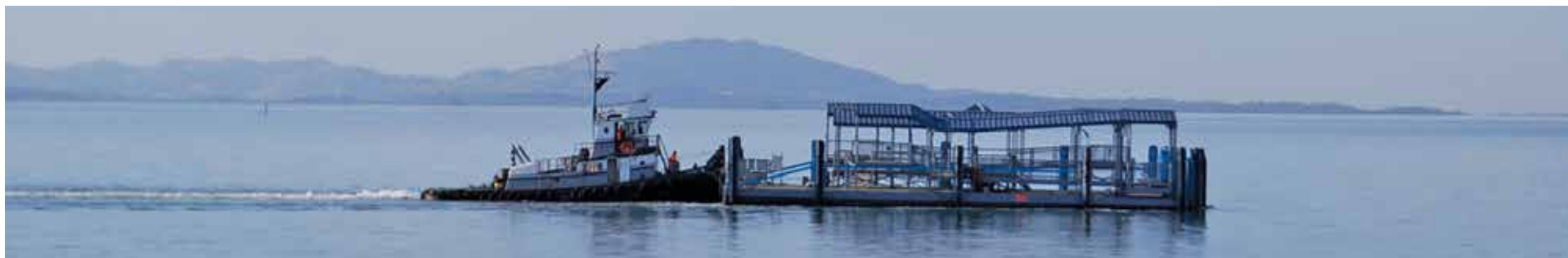
Clockwise from top left: San-Rafael based Dutra Group performs maintenance dredging in the channel leading to the Larkspur ferry terminal. Work continues at the San Francisco ferry terminal to retrofit and replace the boarding ramp cylinders. The passenger float for the Vallejo ferry terminal heads back from Alameda's Bay Ship & Yacht after routine maintenance and upkeep procedures. All photos by Joel Williams
