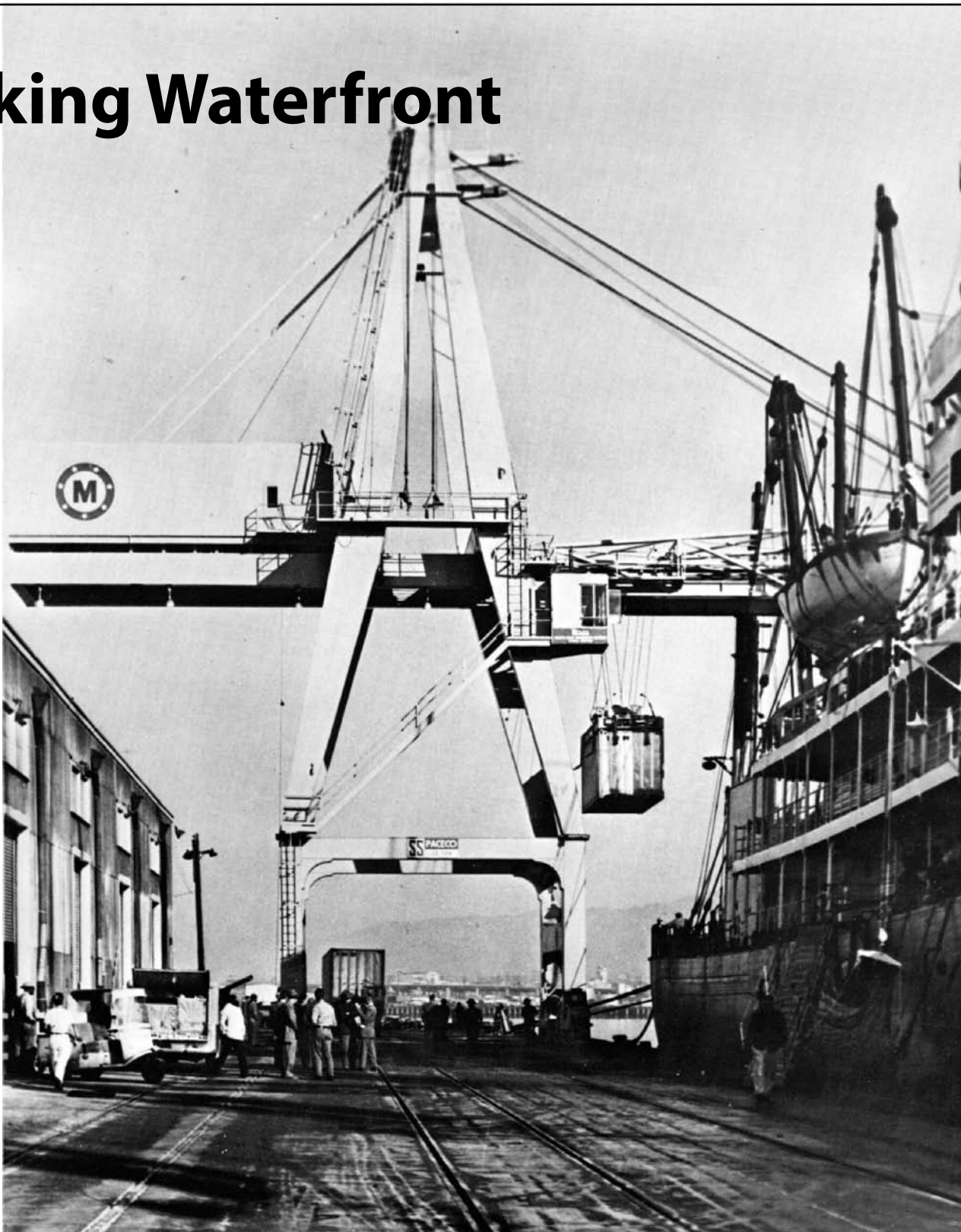
The Matson Encinal Terminal container crane was the first of its kind and a bellwether of the profound change containerization would bring to the world's economy. Installed in 1959, it was moved to China's Port of Nanjing in the 1980s.
