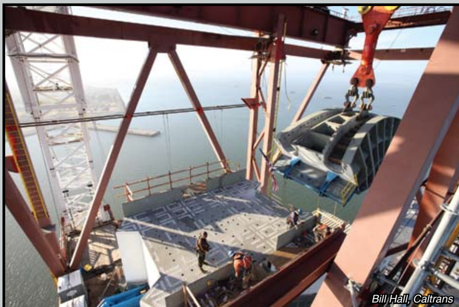
The "world's largest cable saddle" is lifted to the top of the new East Span tower (left) some 500 feet above the Bay. Next, the 450-ton saddle is positioned just above the tower (right), where workers prepare to lower it into place. The signature tower will be crowned with a decorative head once the cable is installed early next year.
