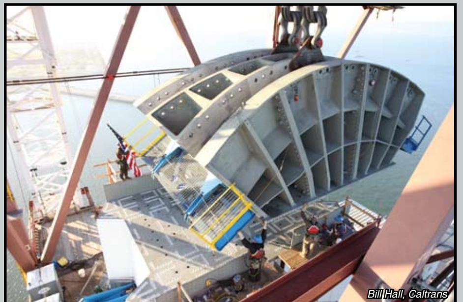
The "world's largest cable saddle" is lifted to the top of the new East Span tower (left) some 500 feet above the Bay. Next, the 450-ton saddle is positioned just above the tower (right), where workers prepare to lower it into place. The signature tower will be crowned with a decorative head once the cable is installed early next year.
