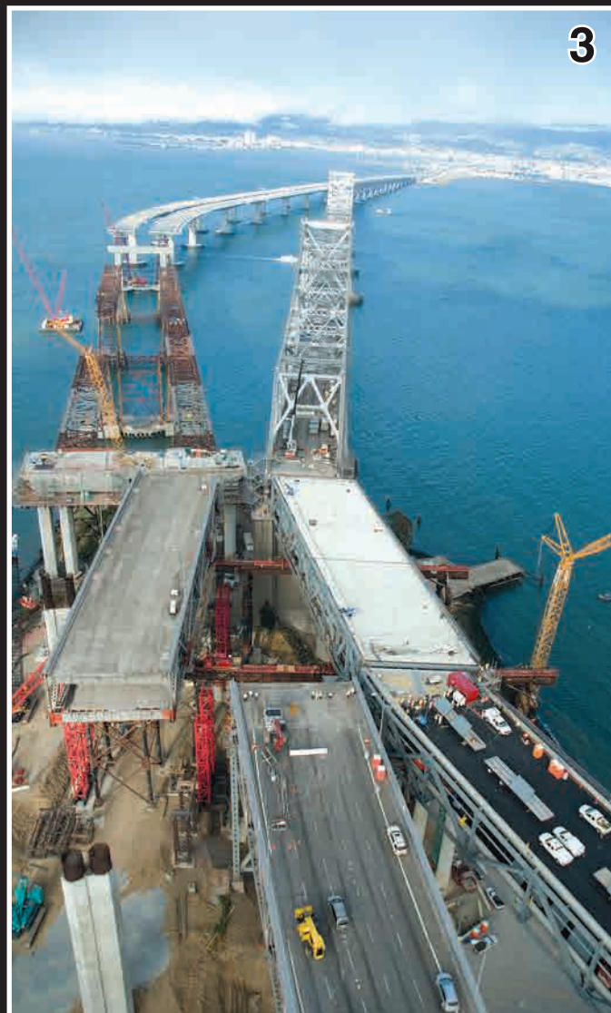
Frame 1: The prefabricated, whitish double-tiered deck section is poised to slide in.
