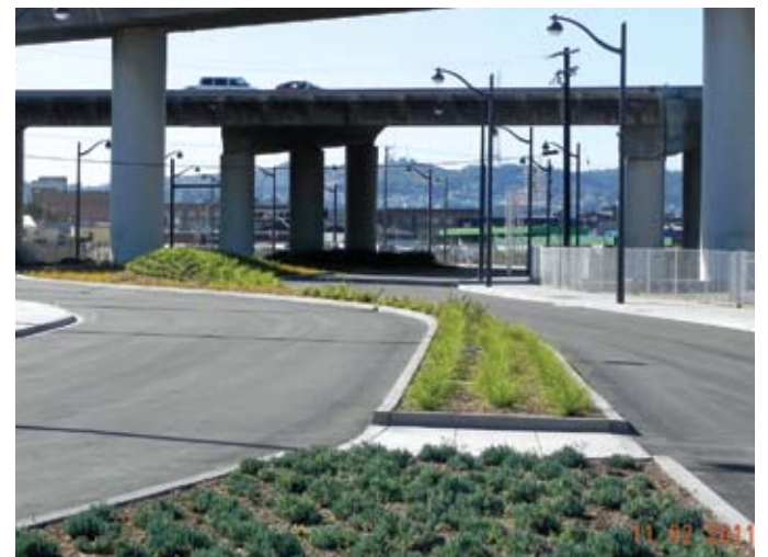
Permeable landscaped surfaces like the Mission Bay Circle will ease the strain on The City’s combined sewer system during heavy rains by absorbing water that would otherwise flow into the sewers.
