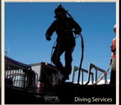
Tracy Boulevard Bridge Seismic Retrofit
