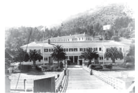
View of the Immigration Station Administration Building from the dock, probably in the 1920s (based on size of palm trees).
