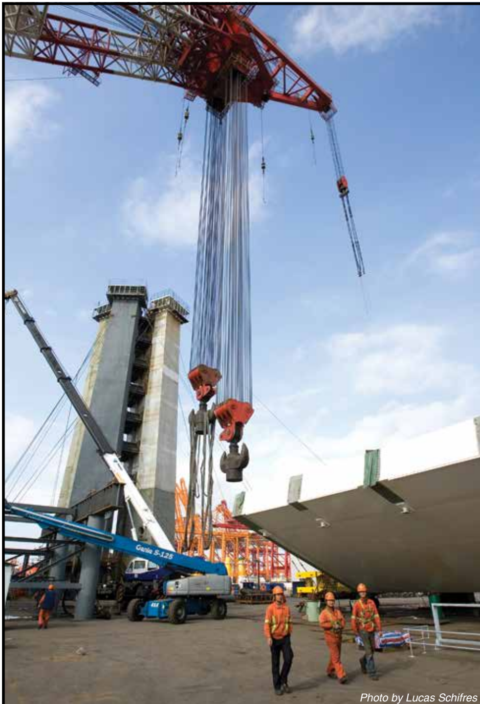
With the first legs of the SAS tower looming in the background, a trio of Team China members stands dockside beside an orthotropic box girder segment ready for shipment.
