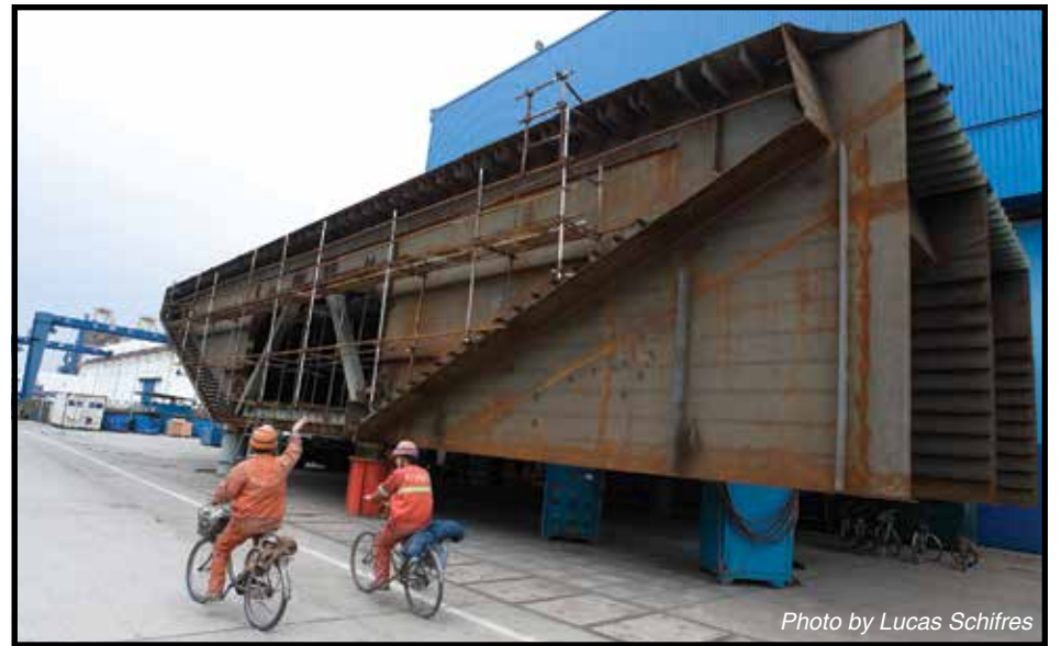
ZPMC workers pedal past an orthotropic box girder section that will form part of the bridge superstructure.
