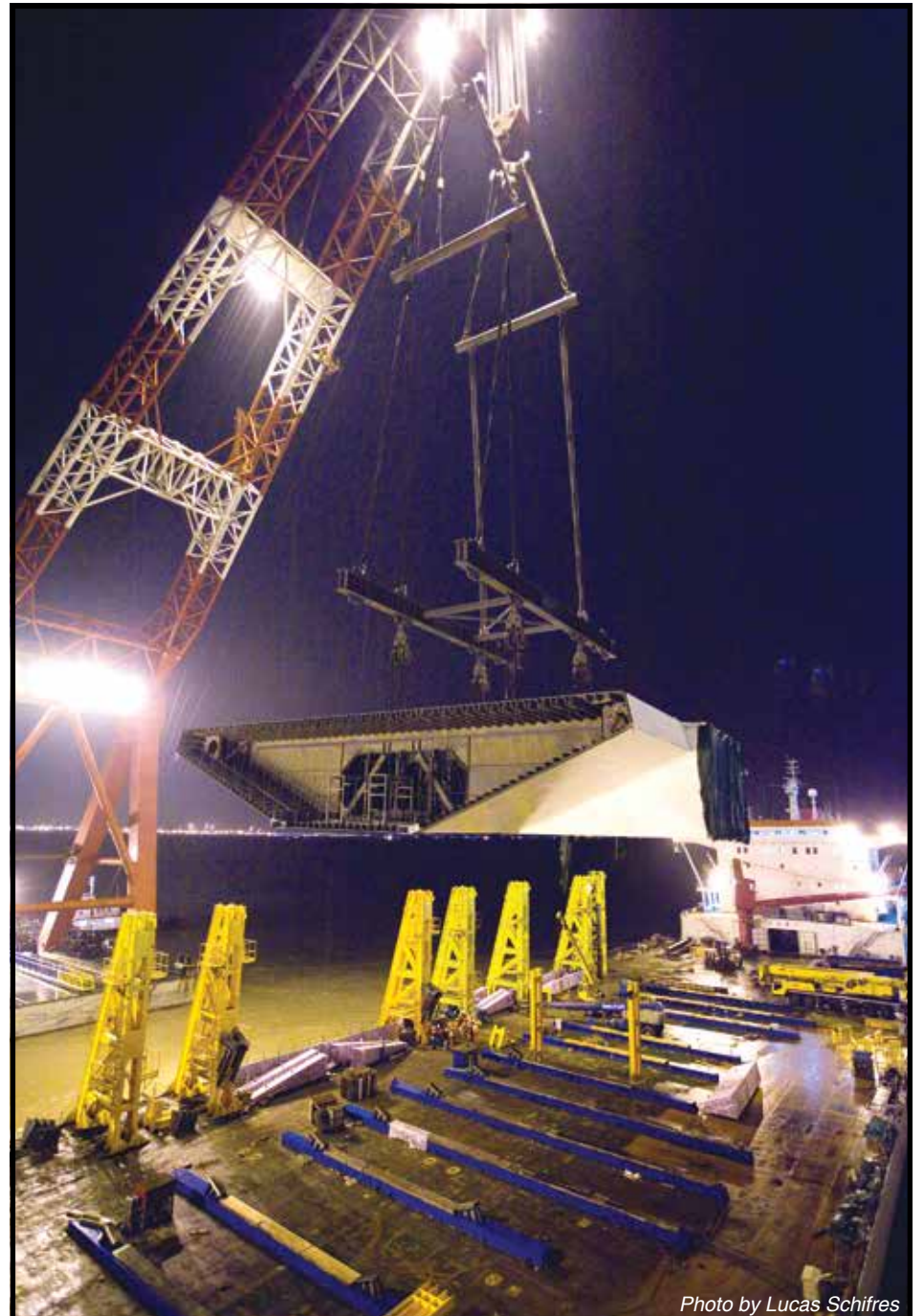
A giant barge-mounted crane prepares to lift a section of the new bridge onto the ship for transport to San Francisco Bay.
