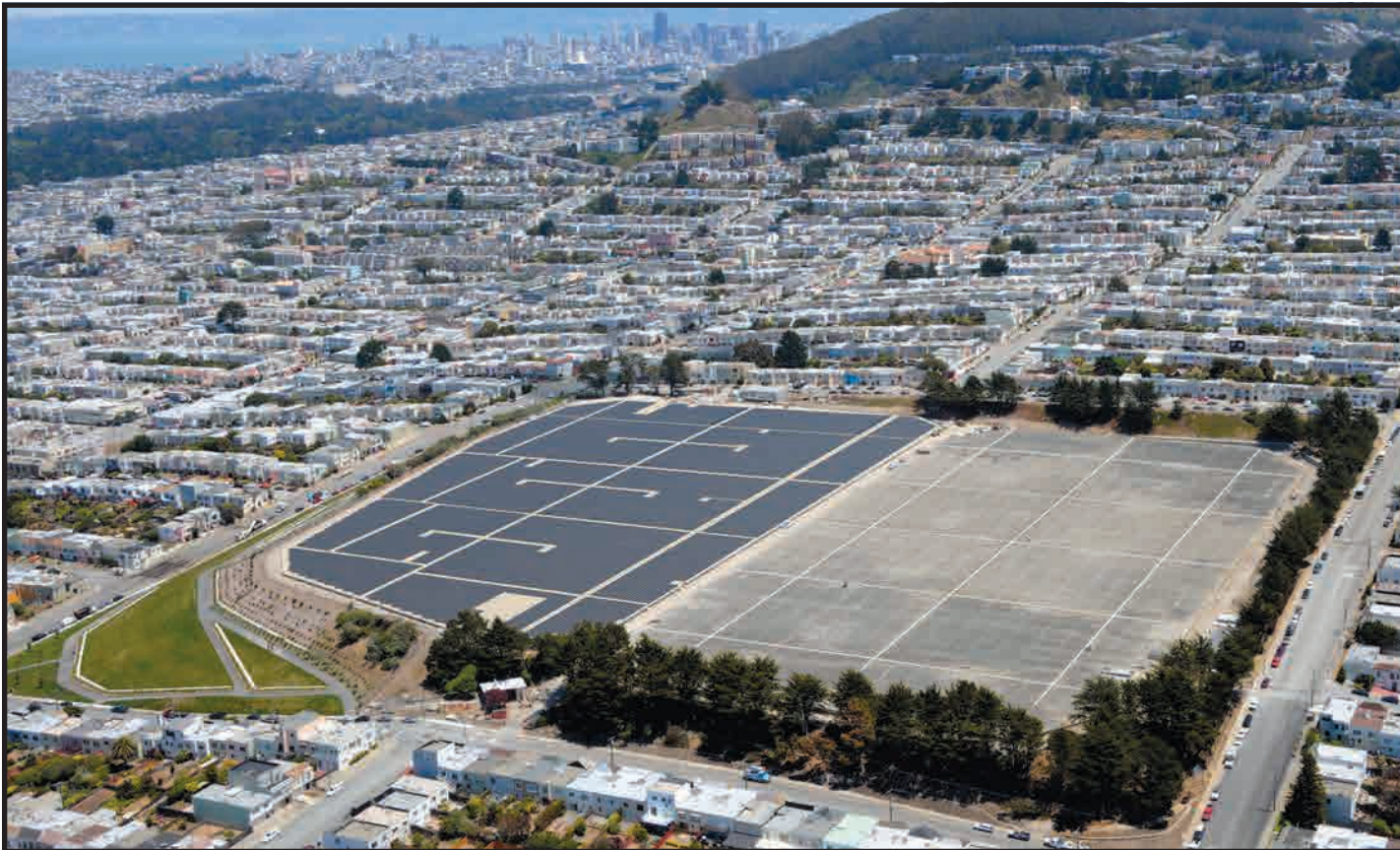
Aerial view of the Sunset District reservoir with an artist rendering of what the planned solar array will look like once installed. Below: From street level the new solar array will be barely noticeable.
