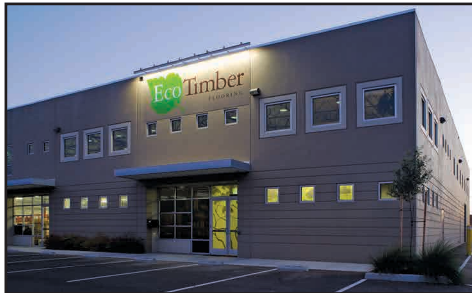
A big reason that EcoTimber decided on the new Richmond location on Central Avenue—sandwiched between I-580 and I-80 just before the roads merge—was the central location in the Bay Area.
