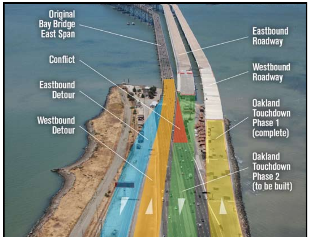
A schematic showing how the detours will allow for the completion of the Bay Bridge East Span touchdown
