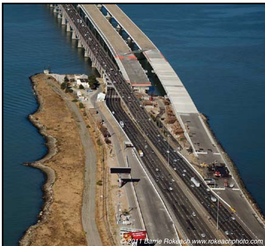
The Bay Bridge touchdown as it now exists, with the twin decks of the new East Span coming in from the right
