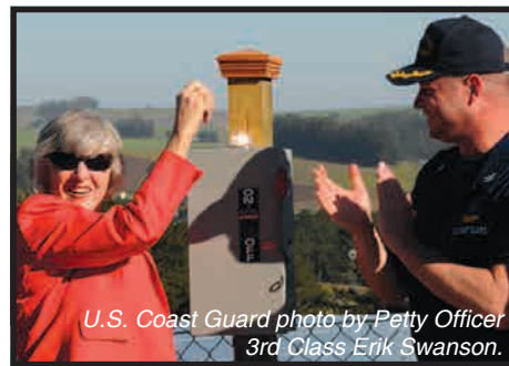
U.S. Coast Guard photo by Petty Officer 3rd Class Erik Swanson. Congresswoman Lynn Woolsey helps Capt. Christopher Hall flip a power switch to signify the opening of the newly constructed solar array field.
