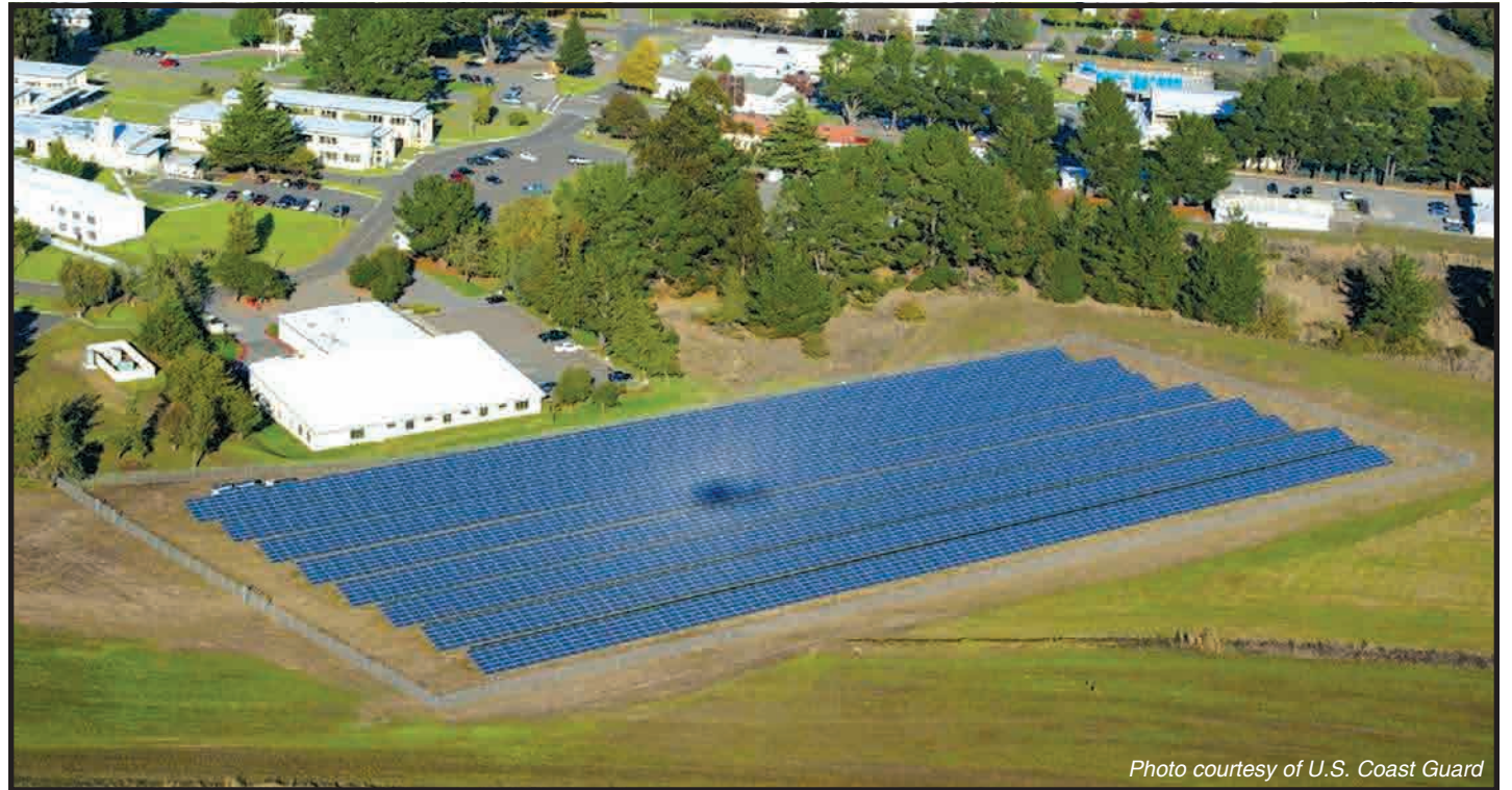
The new four-acre solar array field will produce approximately one megawatt of clean renewable energy each year for the Coast Guard Training Center in Petaluma.
