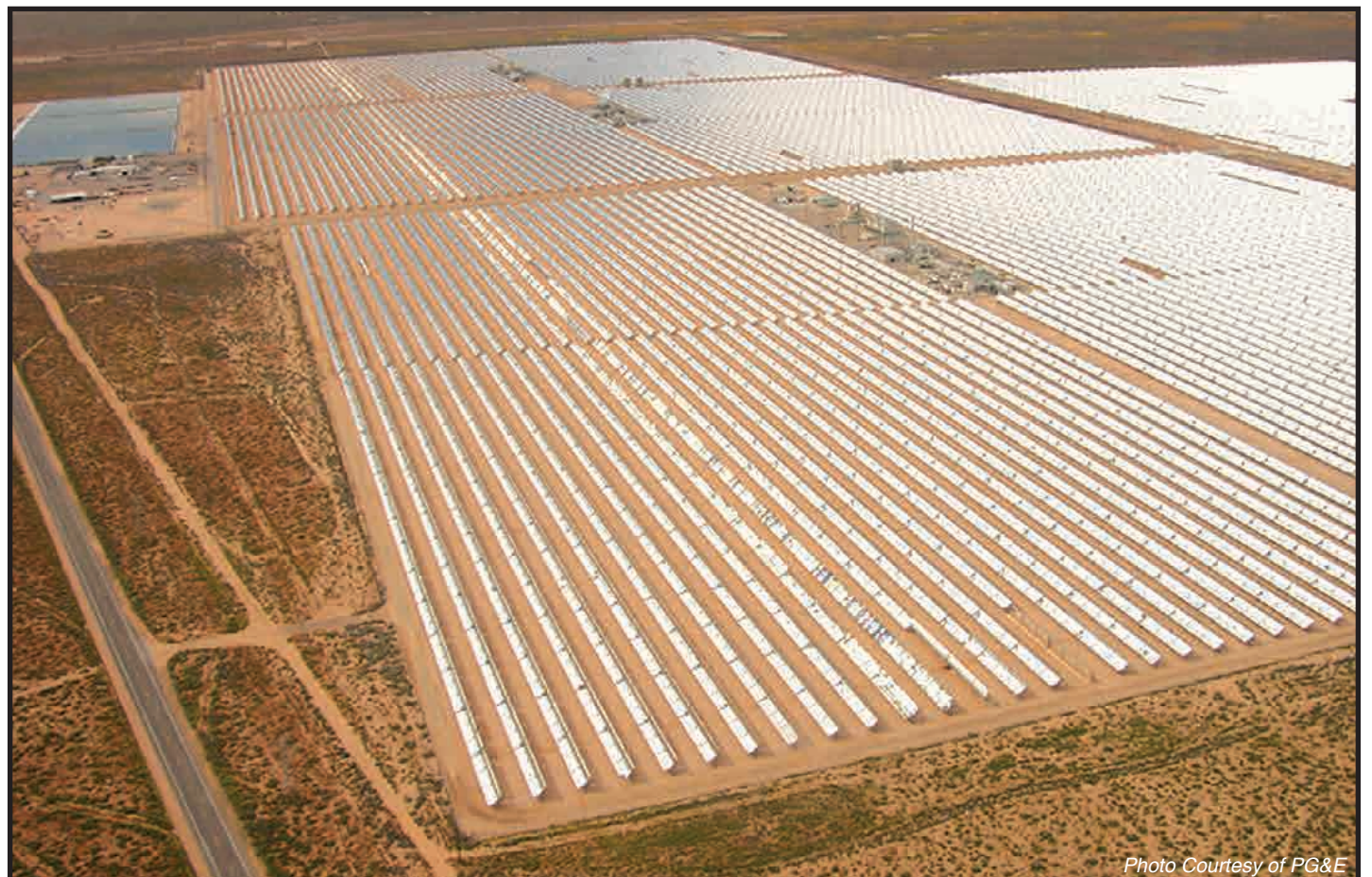
PG&E signed an agreement with Martifer for over 106 MW of renewable solar-thermal biogas hybrid power.
