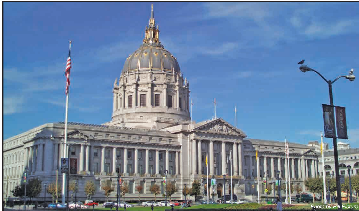
San Francisco's City Hall will be one of the first municipal buildings to get a green makeover as part of the City's partnership with the Clinton Global Initiative to create the country's first green civic center.
