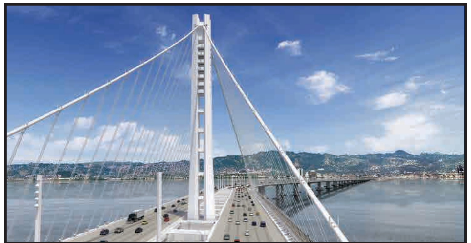
Simulated view of the Self-Anchored Suspension portion of the new Bay Bridge East Span, looking east.
