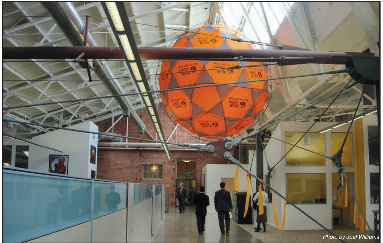
The sawtooth roof at the Ford Point Building features large northern skylights that provide abundant natural light.
