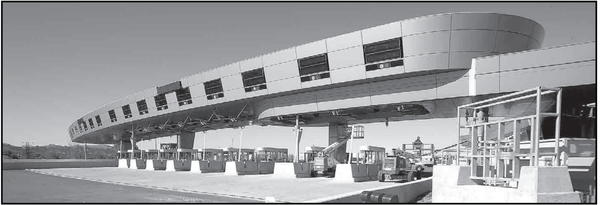
The futuristic toll plaza of the new Benicia-Martinez bridge is designed for open-road tolling, allowing motorists with FasTrak® toll tags to pass through the far left lanes at highway speeds. Photo by John Huseby, Caltrans
