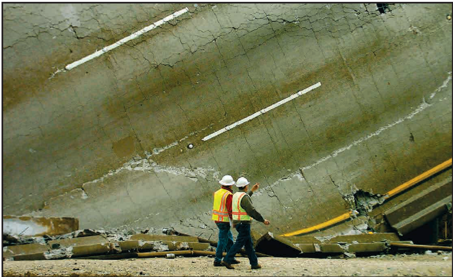
Left: Heat from the tanker accident on the I-80-I-880 connector was so intense that it caused a section of the overpass above – the I-80 to eastbound I-580 connector — to melt onto the roadway below. (Photo by John Huseby, Caltrans) Above: Workers survey the damage. (Photo by Noah Berger) Below left: California Senator Barbara Boxer joined other state and federal officials at a press conference at the Maze site. (Photo by John Huseby, Caltrans) Below right: Caltrans and MTC moved quickly to alert commuters to traffic detours and the offer of free transit rides, with the result that the Bay Bridge toll plaza was virtually deserted the following Monday morning. (Photo by Noah Berger)
