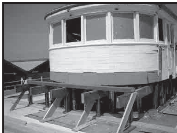
Fresno 's wheelhouse braced for liftoff.
