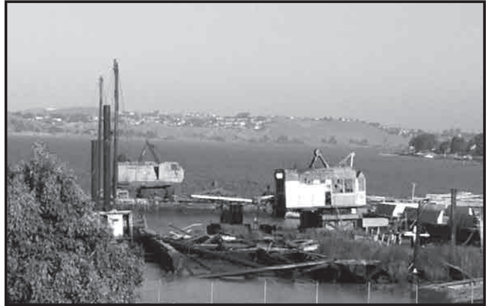
Old Garske ship yard in Benicia about to undergo formidable redevelopment
